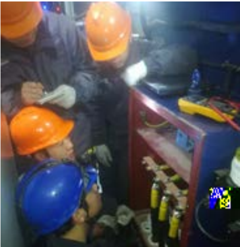
Longyuan Ningxia Company carried out with the goal of "doing a good job in deep maintenance and restoring the performance of the equipment", made an actively deployment in response to the problems, solidly promoted the deep maintenance of wind turbines, and injected new impetus into the company's high-quality development.
